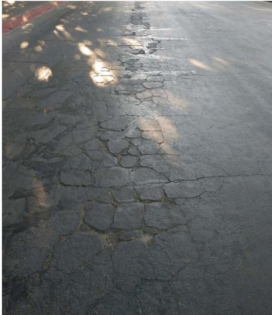
**Figure 12: Fog sealed and striped road rated at 19 PCI (very Poor condition) located on F St in Los Banos.**
