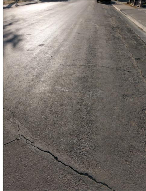
Figure 15: Fog sealed and striped road rated at 81 PCI (satisfactory condition) located on F Street in Los Banos.
