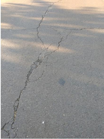
Figure 14: Fog sealed and striped road rated at 71 PCI (fair condition) located on 2<sup>nd</sup> Street in Los Banos.
