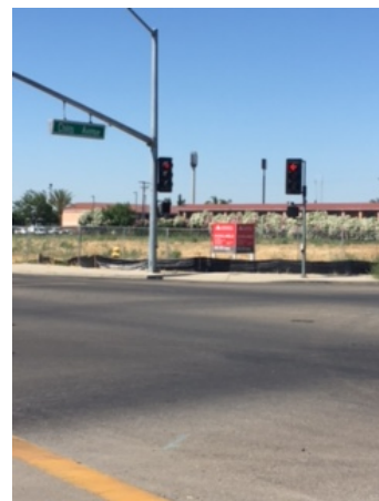
The bowling alley has been demolished and the lot has been cleared and fenced.
