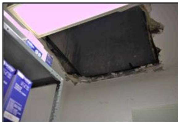
Hole in storage closet ceiling appeared moldy
